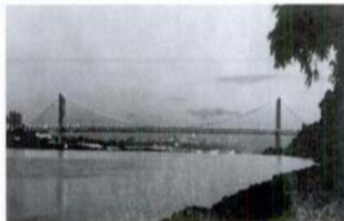
Gambar The George Washington Bridge.
