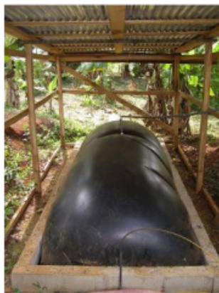
Gambar 4.7. Biodigester Tipe Balloon Plant (Balon)
